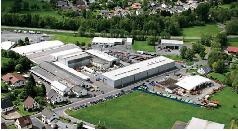
Company premises, Nistertal
